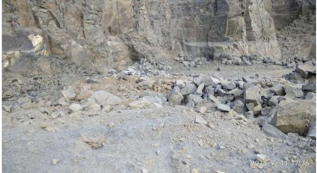
Quarrying detected in expired lease in Ainapura village in Vijayapura Taluk.
